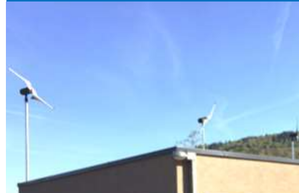
Flange-mounted to a flat roof building
