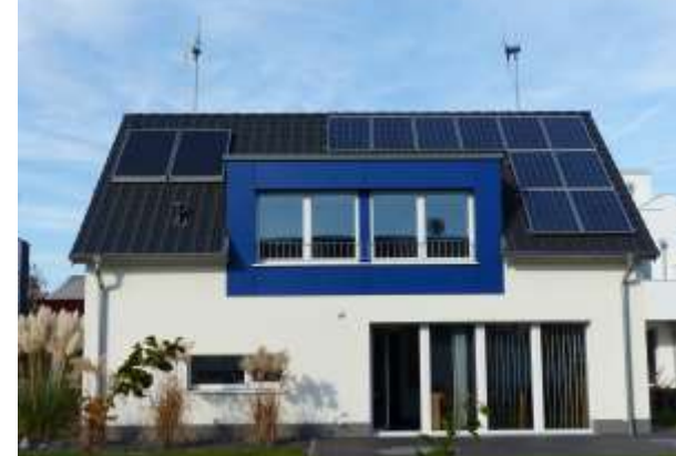
Decoupled towers mounted under the roof-tiles
