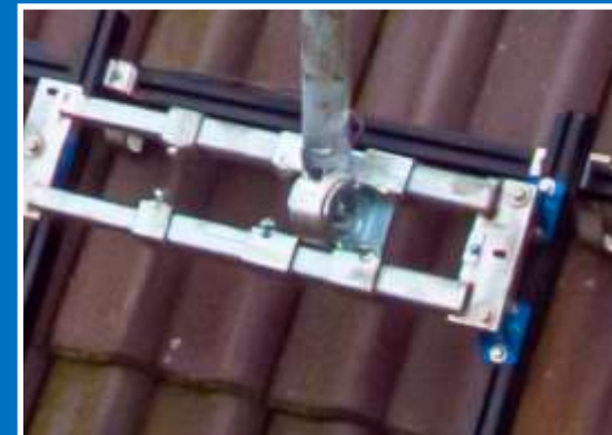
Noise/vibration decouplers (V 15) by ROSTA GmbH of Swiss are maintenance-free and safe
